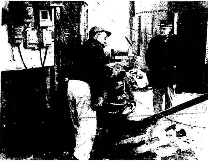
A FLIP OF the switch and 150 head of cattle on the Earl Anderson farm come on the run to the feed bunks. Six minutes later the silage is distributed evenly along the bunk and Mr. Anderson is free to go on with his other chores. An electrical augering system automatically carries, mixes and distributes the feed and the cost for electricity is approximately eight cents a day.
