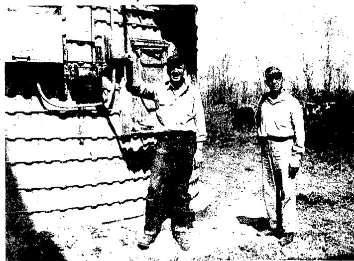
THREE-PHASE USERS of electricity are cropping up throughout the district. Glenn and E. W. Lundahl are two of the latest farmers to put this type of power to use on their stock and grain farm east of Wayne. This type of installation provides steadier power with maximum efficiency and allows the use of lighter weight motors. The
